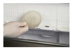
4. Remove the plastic cap & spring located on the bottom of sump/freezing chamber to drain out all water and scale deposits. (On the AC/EC 206 & 226 remove the plastic sump cap in the storage bin)
