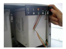
2. Remove the front unit panel & evaporator cover so to gain access to both the water sump area and the evaporator section.
