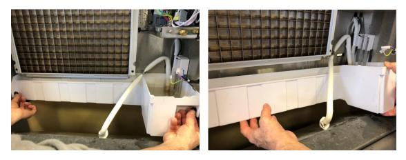
Using a prepared solution, rinse and wipe down the sump chamber.
