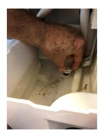
OR, turn the unit on with the water supply isolated.
