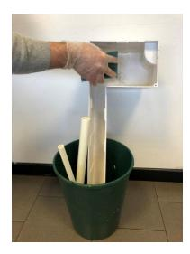
All above steps should be completed using an approved antibacterial solution (finally rinsed by fresh water) then, carefully re-assemble all removed parts.
